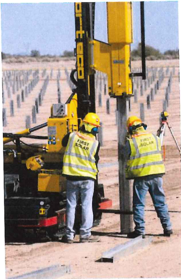
Photograph 3: Installation Process – Posts Driven into the Ground Surface to Support PV Modules at a Solar Energy Generating Facility
